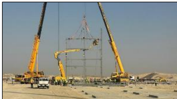
Figure 8 Pre-Assembled structure during installation
